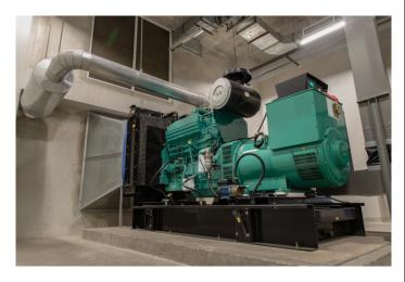
Everyone knows that the emergency generator has to be inspected and tested, however the details on how to conduct the inspection and test is where the gaps usually appear. For example, the monthly generator test must be at 30% of the nameplate rating of the generator or reach a specific exhaust gas temperature.
