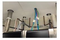
pipes. Staff performing the above the ceiling work need to be educated on the need to seal these gaps and again an inspection process after the work to verify the work was done in a compliant fashion.
