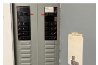
opening electrical breaker boxes and looking for any "spare," unlabeled breakers that might be in the on position. If the spare, unlabeled breaker is on, chances are it is actually providing current to some part of the hospital or equipment. Thus, the organization has failed to properly label its utility shut offs.
