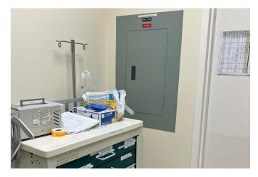
It could be as simple as blocking electrical panels. Commonly it can also be open junction boxes that contain live wiring, where someone has left the cover off. It may also be that you are missing battery powered task lighting for the generator that an operator may need if the generator has failed to start.
