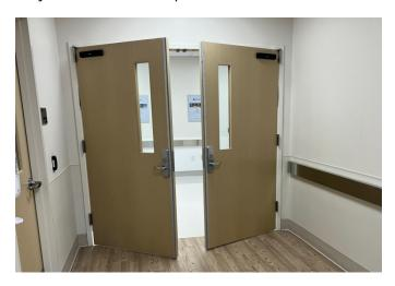
The article then details the requirements for fire resistance ratings on those smoke doors or fire doors. Smoke doors for new construction built or plans approved after July 5, 2016, must have a 1-hour fire resistance rating. These smoke doors must be self-closing or automatic closing but are not required to be self-latching.
